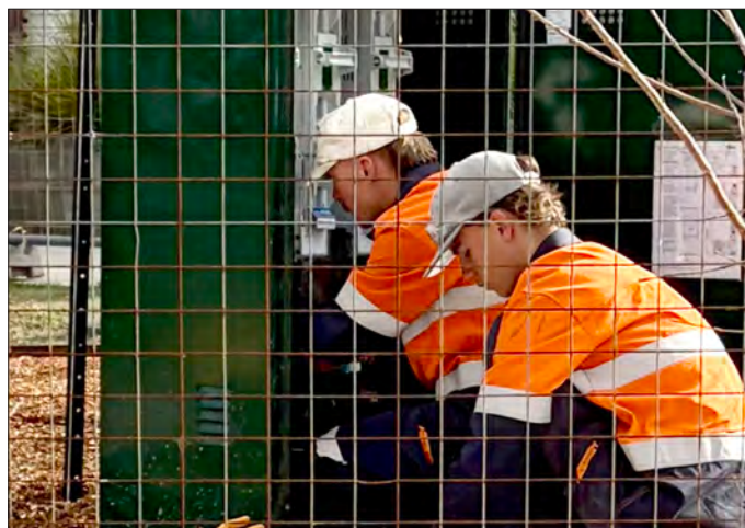
Connecting to the main grid. Photo: John Walters
