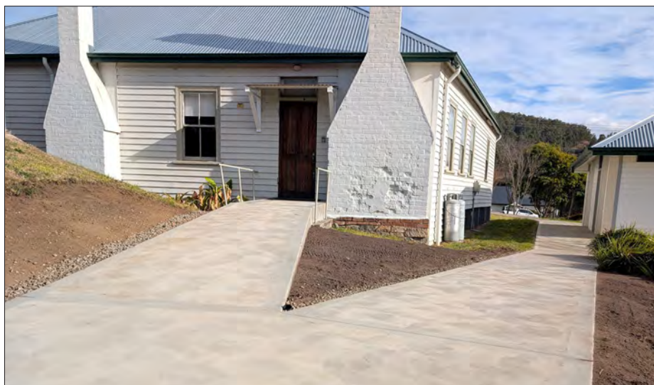
The new disabled access ramp from the disabled parking area to the back entrance of the hall, giving access to kitchen, supper room and the stage.
