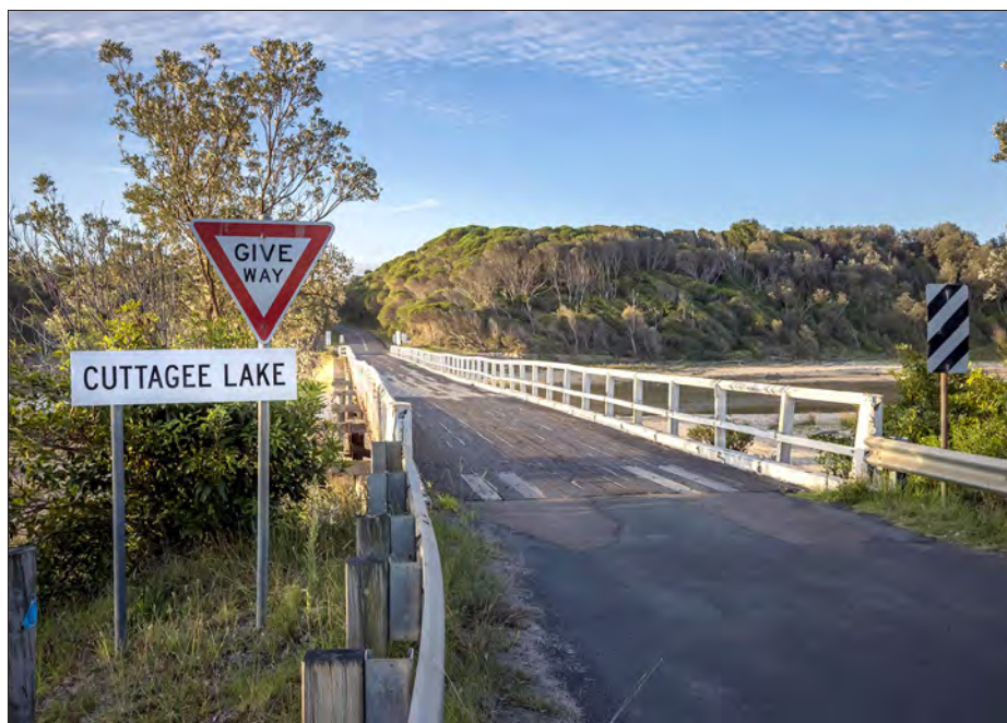
Cuttagee Bridge David Rogers photography
