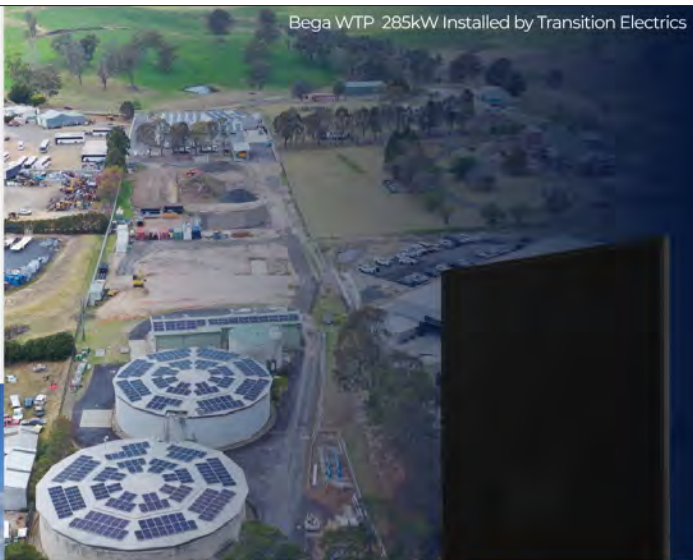
Bega WTP 285kW Installed by Transition Electrics
