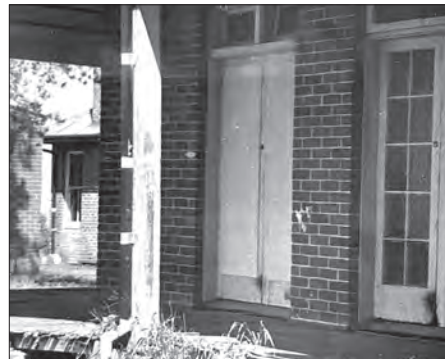
Old Bega Hospital before renovation
