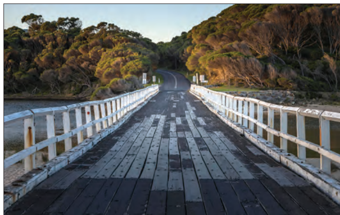
Cuttagee Bridge Photo: David Rogers Photography
