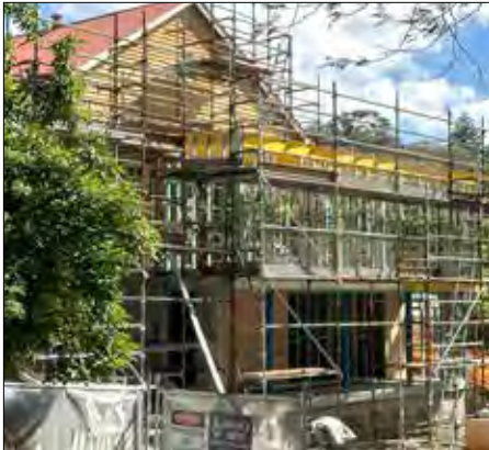
Scaffolding at the Halls
