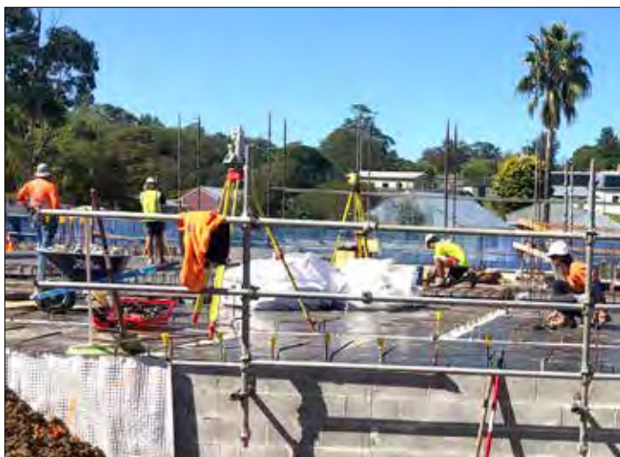
The eastern site – after the concrete pour.
