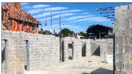
The basement of the market hall
