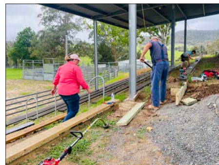
Simon Cooke installing new seating and Leanne Salway prepping to paint.
