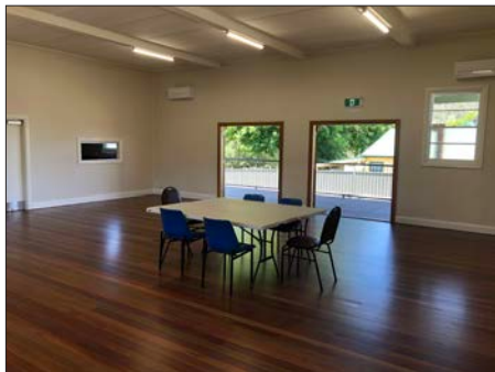
The refurbished RSL Hall ready for a new life serving the RSL and the community Photo: John Walters
