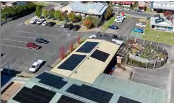
Drone image of the solar panels on the roof of the Cobargo Co-op.
