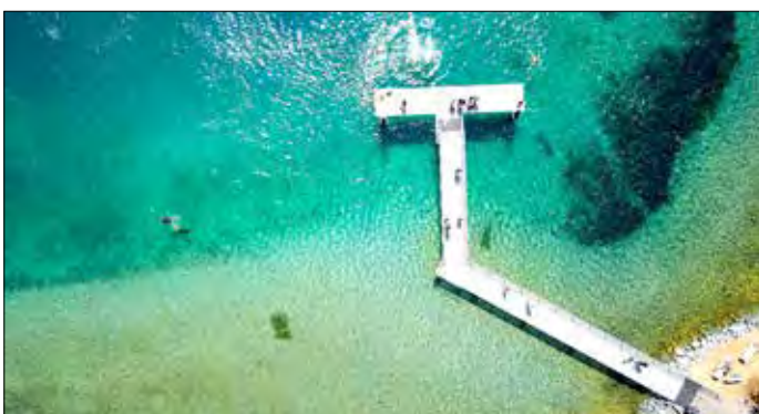
Aerial view of the new jetty and pontoon
