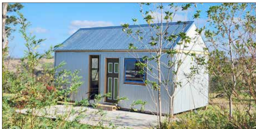
The '50 sheds' project is a collaboration between the Triangle Tool Library and local carpenter Nathan Thompson with support from Vinnies and Anglicare. So far 13 sheds have been built through four households teaming up and committing 16 days. Each 7.2 x 3.6 m pine framed and tin-clad shed with a gable roof takes four days to construct and costs about $10,000 in materials to basic lockup. Interested in one of these? Contact Monica Considine: monica.considine@gail.com
