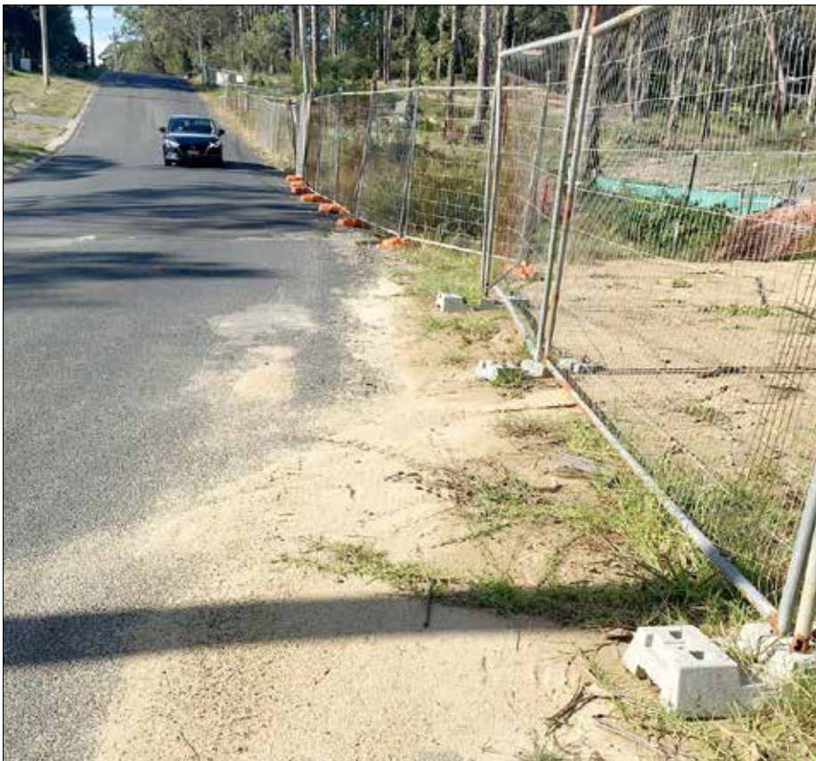
The builder's exclusion fence impinging on the roadway but failing to prevent sediment running off into Wallaga Lake.
