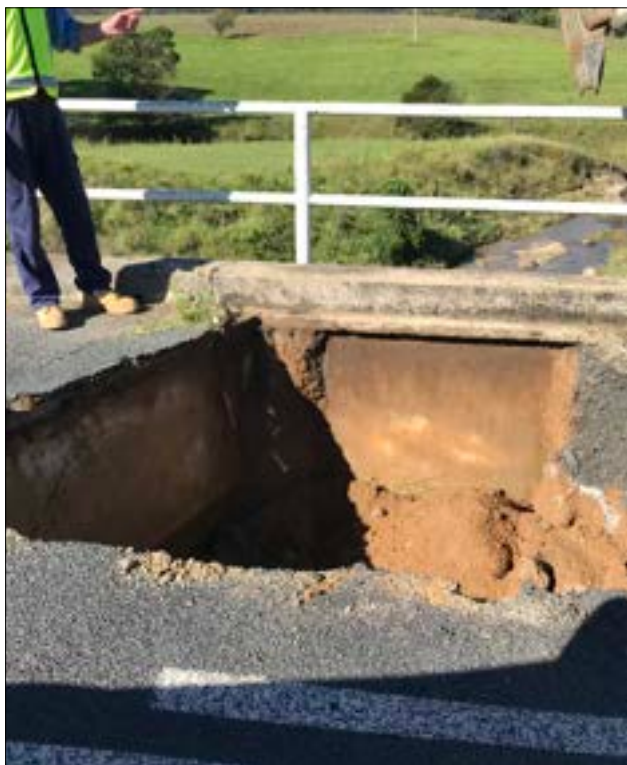
After eighteen months of heavy traffic and ten days of rain, Wilgoa Bridge, on Wandella road, developed a huge hole that was speedily rectified by Council. Photo credit: Louise Brown
