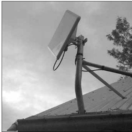
A rooftop NBN fixed wireless antenna
