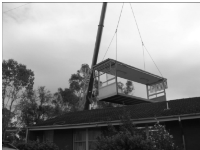
Huge cranes were used to swing in the new sections and remove the old demountable classrooms..
