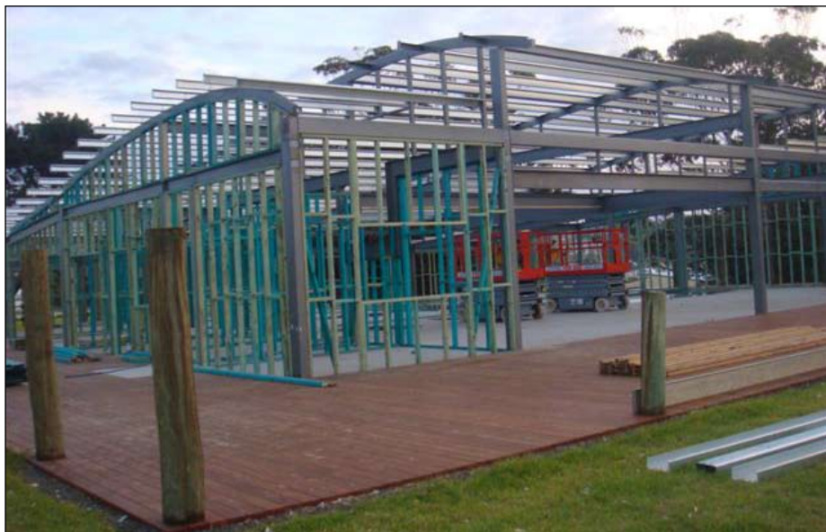
The steel framework goes up for the Bermagui Surf Club's new building
