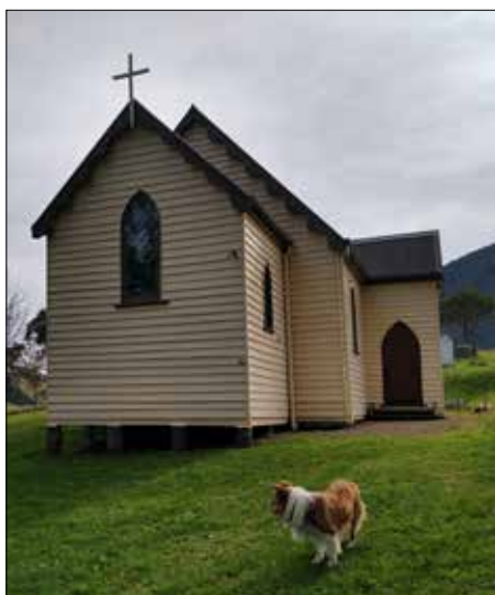
Open Sanctuary, in need of repairs – come along and contribute a gold coin on 3 or 4 October.
