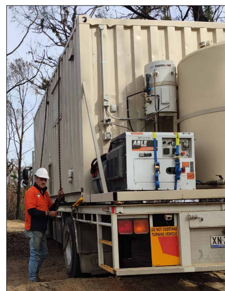
Mal James of Minderoo Foundation gets hands-on with pod installation at Stefan's place.
