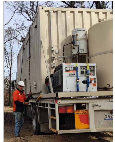
Mal James of Minderoo Foundation gets hands-on with pod installation at Stefan's place.
