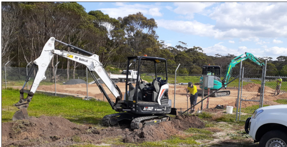
Sods are being turned! Work starts on the Bermagui Men's Shed on the Bermagui-Tathra Road.
