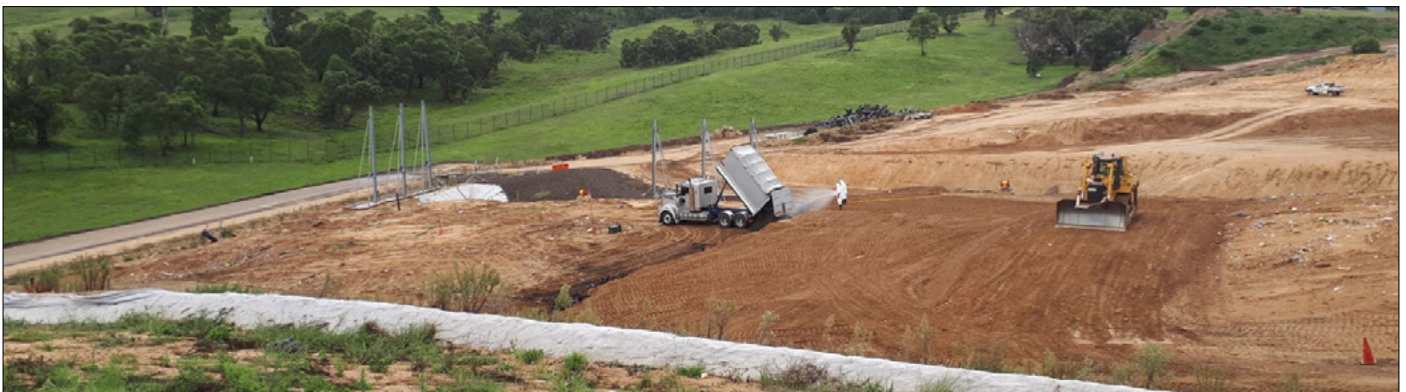
Contractors managing asbestos contaminated fire material into existing landfill at the Central Waste Facility.
