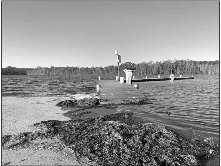
The pier off Regatta Point—the first 'asset' that goes under when the Lake rises
