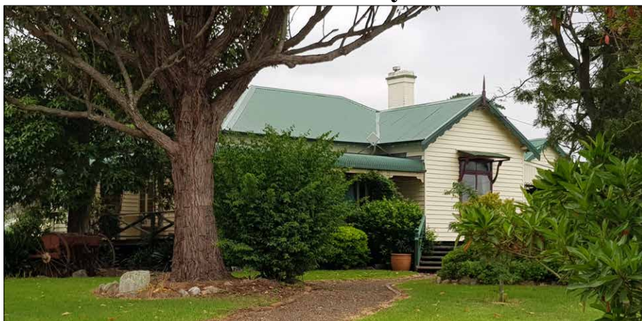
The historic homestead was destroyed.
