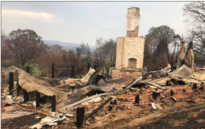
Fire destroyed several of our town's oldest homes
