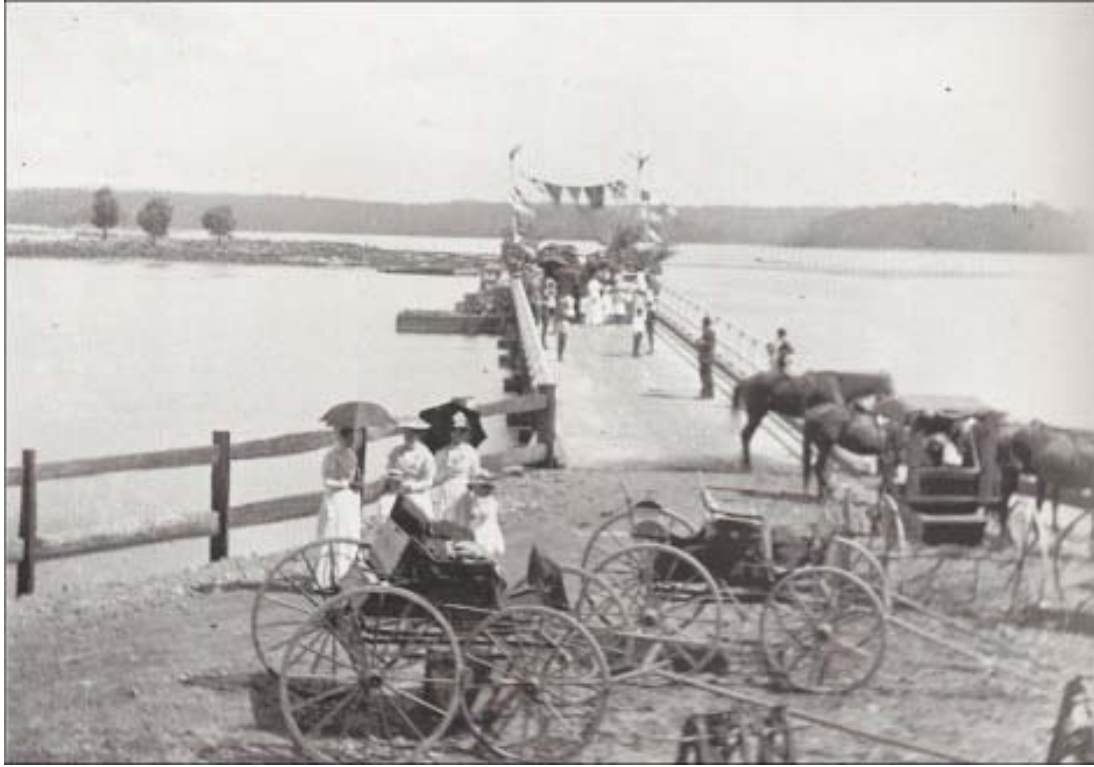
Wallaga Lake Bridge Opening 1894. Photo from the Corkhill Collection, National Library of Australia
